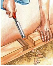
the foundation skids with series of saw cuts, then and toenails (center skid).
