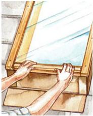
Cut the horizontal flanges of the bottom piece of skylight flashing and wrap the ends around the frame sides. Lay the glass into the skylight frame and secure it with redwood stops. Use a beveled stop for the bottom piece.
