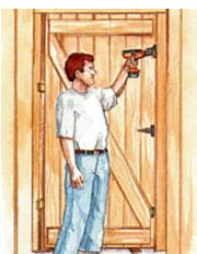
Attach the outer window stops, with the beveled stop at the bottom. Nail the center stops to the mullion. Use shims to set the gaps along the door edges, and mount the door hinges with galvanized screws.
